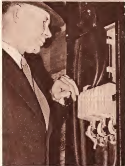
The infra-red lights, as shown in this picture, are strung between the trees and turned on and off thermostatically. Below is the master switch box of a ten-acre grove which has been protected for two years by infra-red illumination. The infra-red light is also believed to stimulate the growth of the trees.
